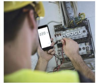
Electric Power Inspection
